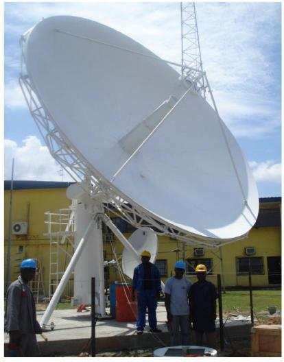
**SilverSatcom** 7.3m antenna exceptional performance makes it an excellent choice for all applications. incorporates stretch - formed doubly contoured panels with matched radials and hub for ease of field alignment provide an accurate surface contour, and extraordinary gain .
